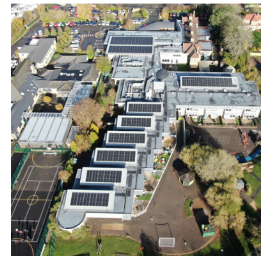
Solar rooftop scheme at Three Ways School, Bath
