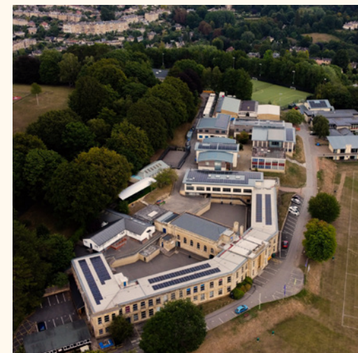
Solar rooftop scheme at Beechen Cliff School, Bath
